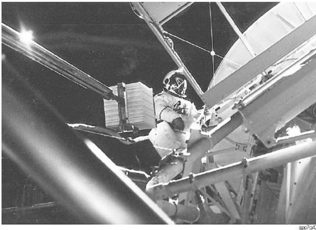
Figure II.2-6.- Powered extendable boom cargo transfer concept.
